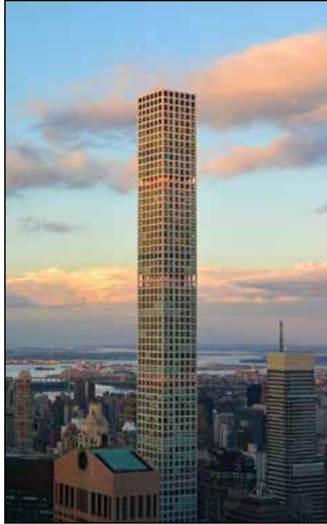
432 Park Avenue has 85 stories above ground: a mezzanine and 84 numbered stories. Five two-story windbreaks, spaced every 12 floors from the top, are unenclosed and serve to reduce the tower's wind load. Photo Credit: Wikipedia
